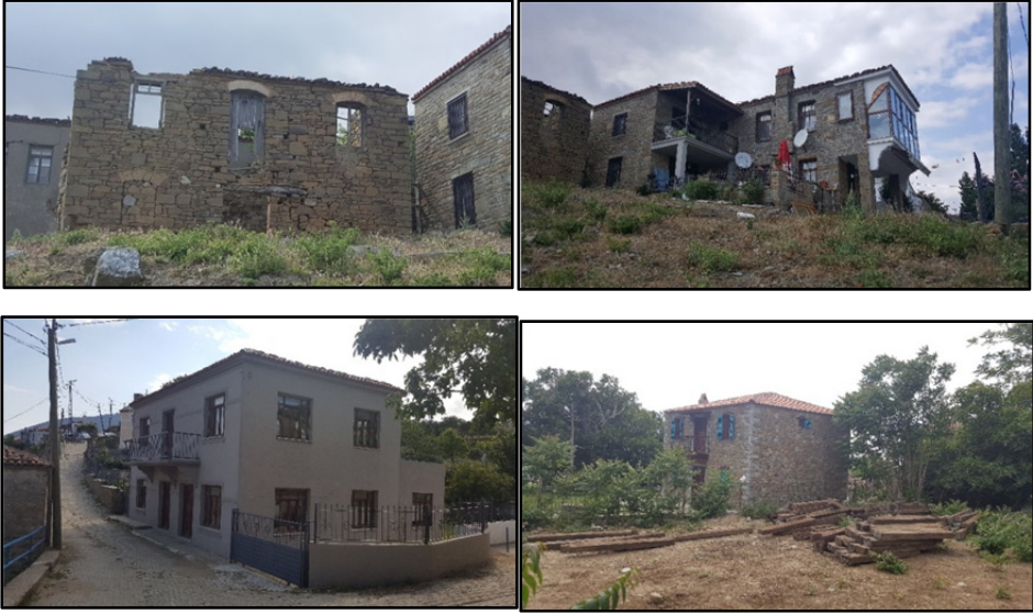
Figure 5. Architectural character of vernacular houses in Gökçeada (by author, 2017)
