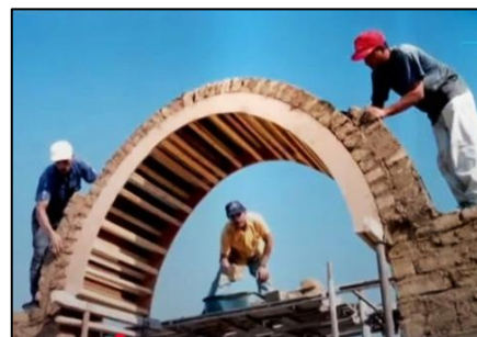
Figure 3. Traditional arch construction at GAV.
