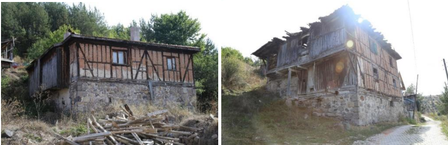
Figure 5-6. A 2-story and 3-story Traditional house in Berçinçatak Village, Kızılcahamam.
